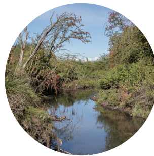
Works to improve the Yeading Brook in Ruislip
